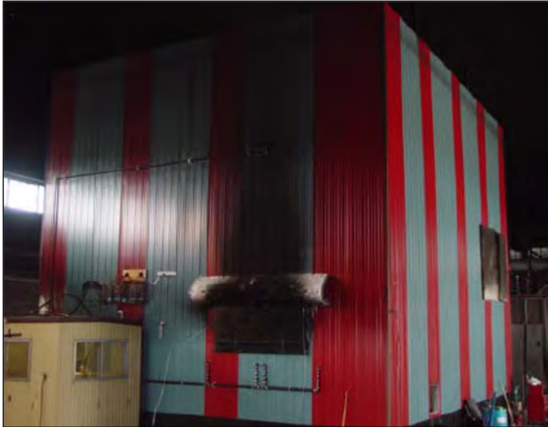
Plate 2 – External layout of the test facility [69]
